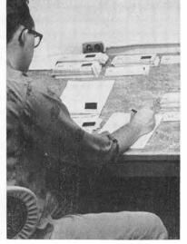
IN FINAL STEP, William Lewis gets 35mm IBM window cards ready to go to Copy Flow. The IBM cards will also be sent to microfilm banks located throughout Sandia Laboratory. At these locations, employees use printer-reader machines which magnify negative 15 times. Quick copies can be made of this size on printer-reader.
